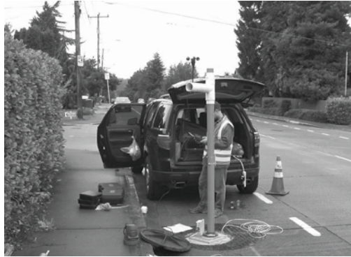
Upstream manhole at North Seattle.
