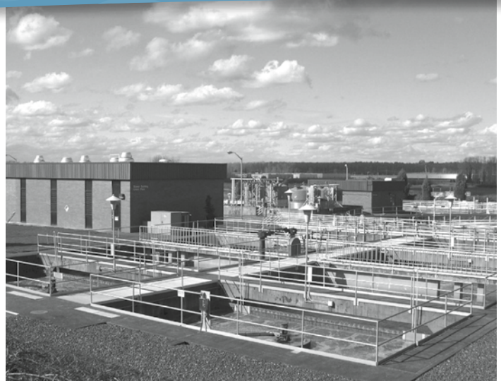
Gresham Wastewater Treatment Plant.
